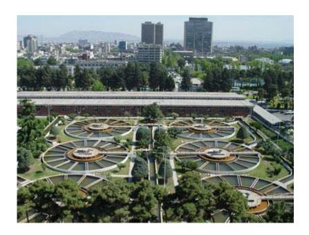
One of the oldest water treatment plants in tehran, founded in 1954. The water is supplied by *Karaj* river, and is transferred to the plant through 2 steel pipes with deiameter of 1000 mm, and length of 40 km.
