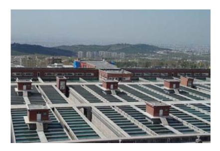
Founded in 2003, water source is *LAAR* damn, water is transferred to this plant through 40 km pipes with diameter of 3600 mm. In this plant water is treated through physical and chemical processes. The 5th water treatment plant of Tehran is equipped with the best Process Control technologies, all parts of plant, valves, elctro motors, gates,... are controlled by PLC system.
