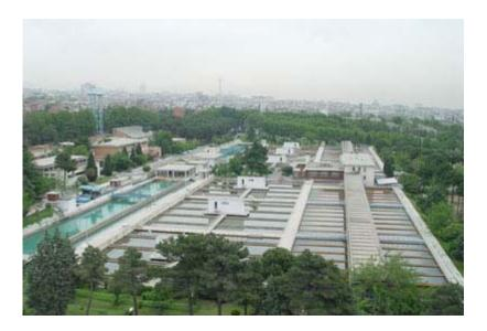
The Bigest water treatment plant of Iran, founded in two phases betwenn 1962-69. The water is supplied by *Karaj* river, and is transferred to the plant through 2 concrete pipes with deiameter of 2000 mm, and length of 33 km.
